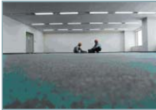
A finished AIS ACBP Type Access Floor with Tile Carpeting Finishing
