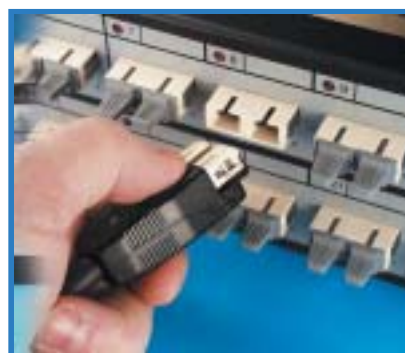
Fibre optic patch panel
