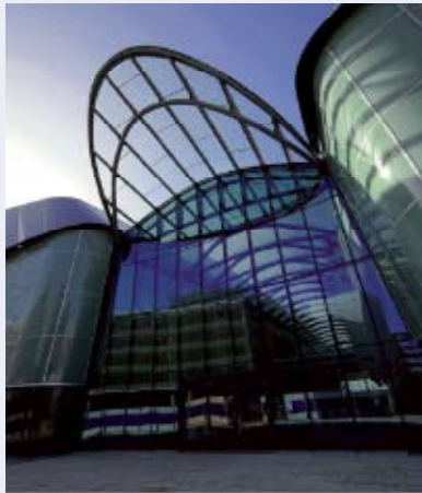
The Liverpool Galleria & Conference Centre
